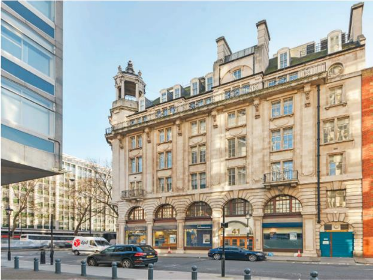
View from Kemble Street
